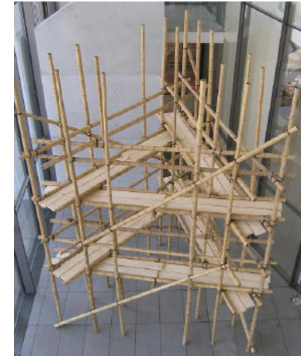
This project is a tribute to Chinese scaffolding, which is built entirely of bamboo. It can be made to reach extreme heights of up to 80 stories and its appearance is handcrafted. They are very stable and are easy to assemble.
